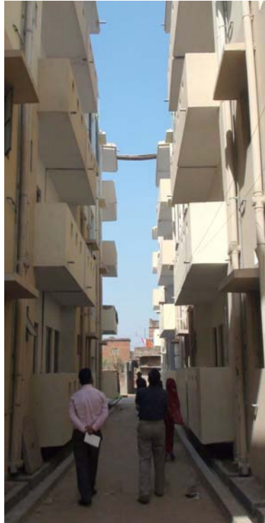
PATNA BSUP REHAB CONSTRUCTION
